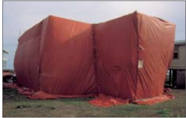
Figure 10. Covered structure fumigation.
